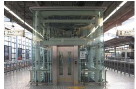
▲Elevator installation (Kyoto station)
